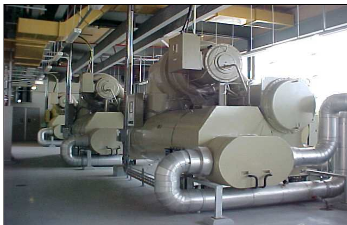
Figure 9: Trane 4.5 MW Water Chillers used for Air Conditioning (N + 1 configuration)
