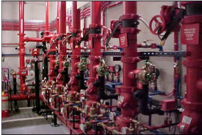
Figure 10: Dry Pipe Fire Suppression System is used in addition to Inergen® Gas System
