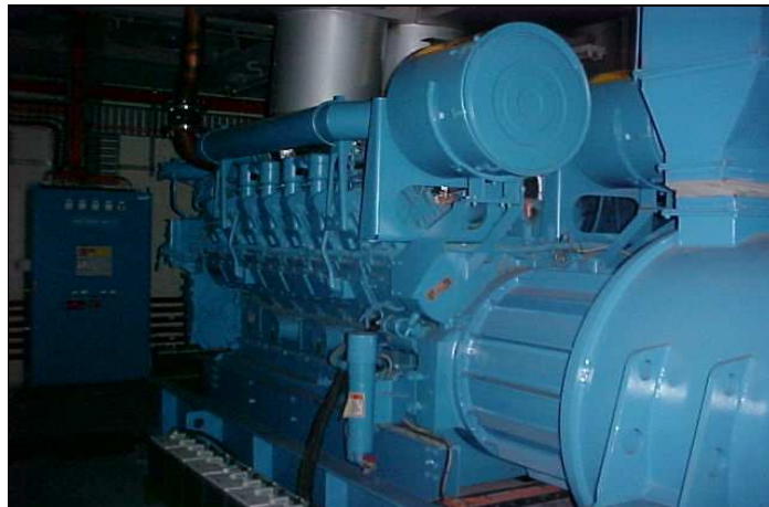
Figure 8 - Caterpillar 2.2 MVA Backup Generator (10 now installed in N + N configuration)
